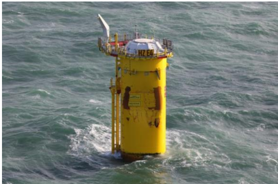
Fig. 1a. A 37200-tons rudderless cargo ship drifted into the Hollandse Kust Zuid wind farm (Dutch North Sea)
